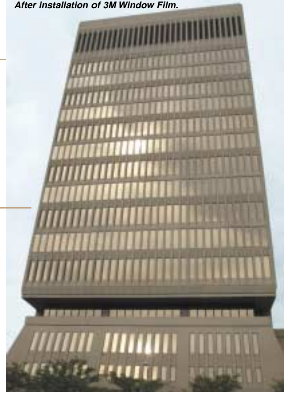
After installation of 3M Window Film.
